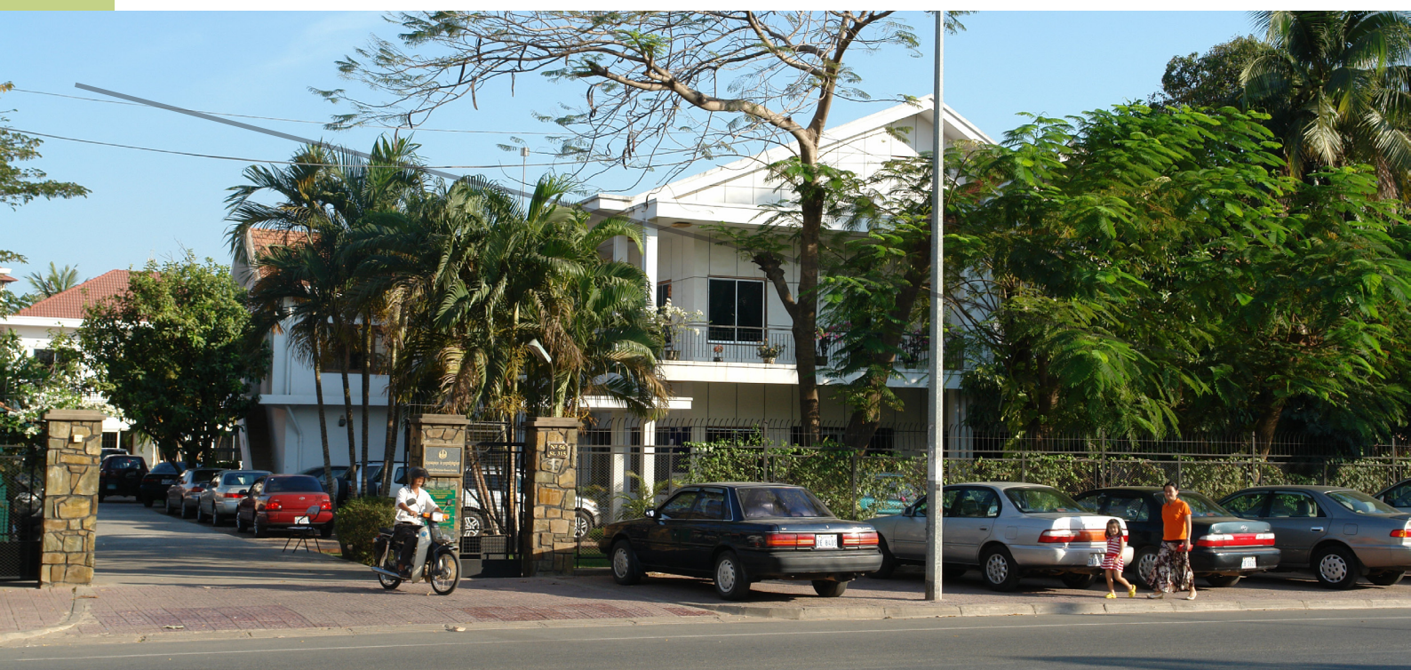
CDRI main building, March 2010
