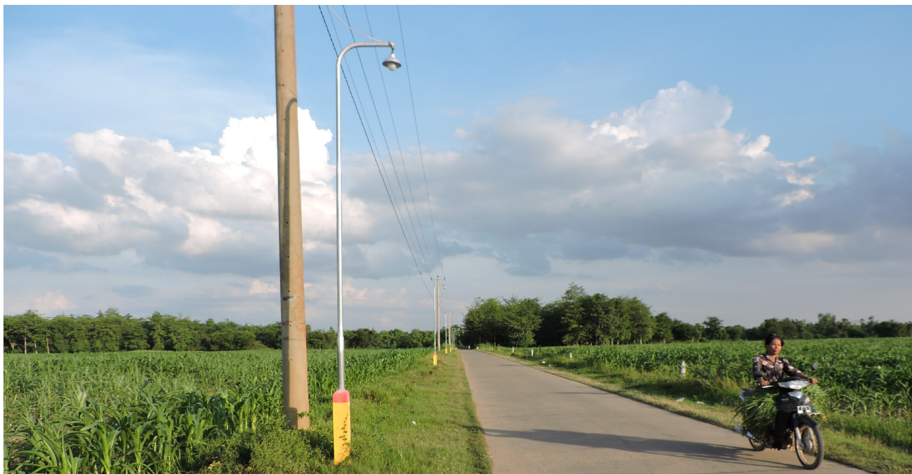
Road improvement continues unabated, with the widening and/or upgrading of many more laterite roads, Kampong Chhnang, Mar 2020
